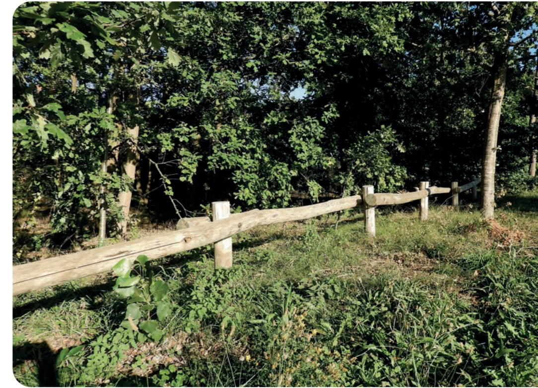
All horizontal beams are finished and predrilled.
